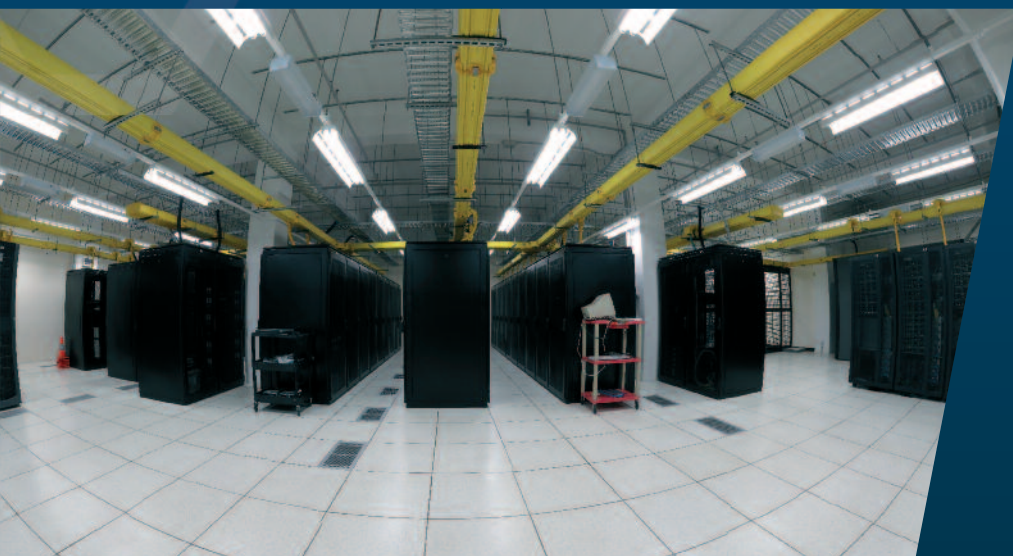
Data Centre – Courtesy of Bob West (CC BY-NC-SA 2.0)
